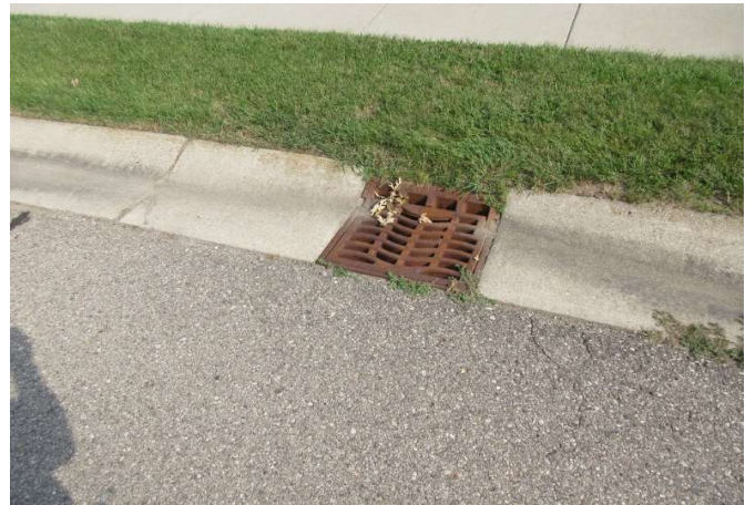
Catch basin in curb
