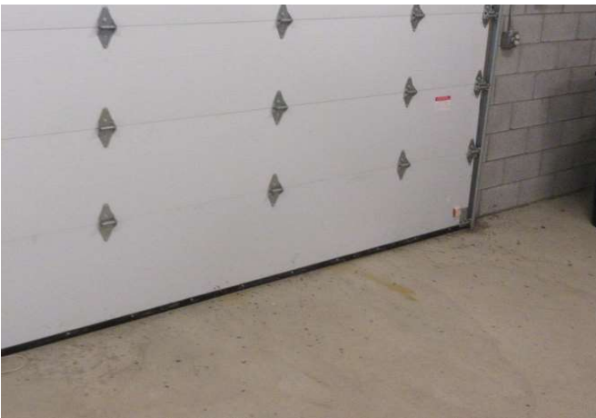
Interior side of panels
