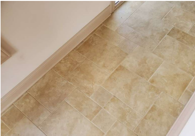
Tile in hallway
