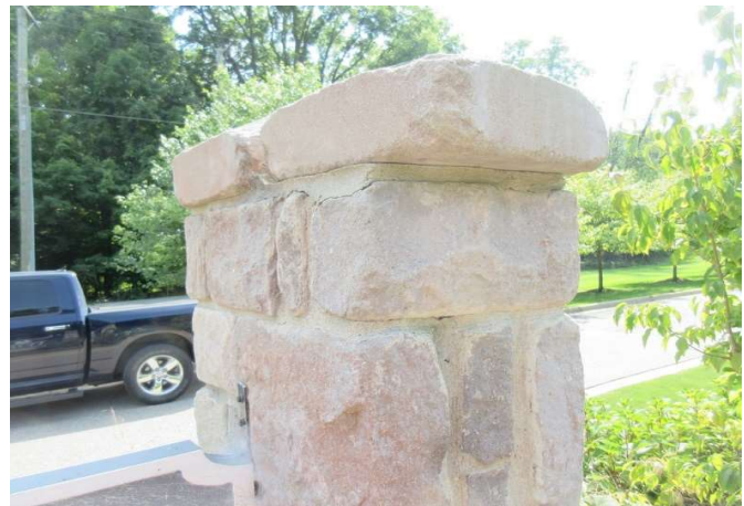
Surface of masonry
