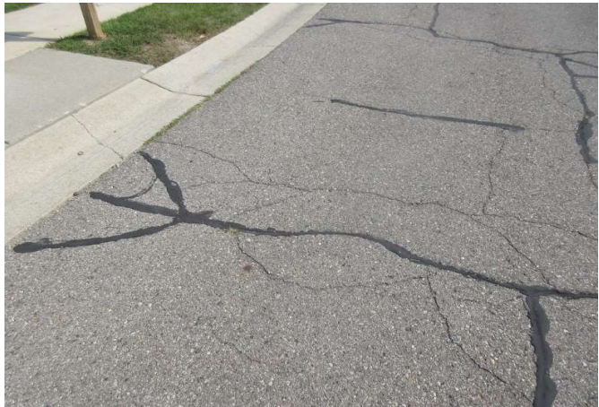
Typical street condition
