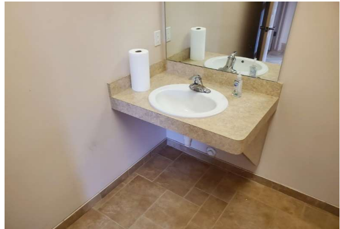
Sink area, typical
