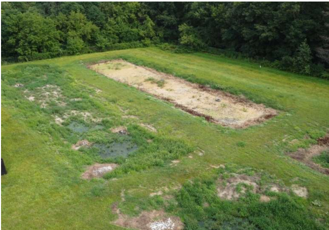
Overview of leach fields
