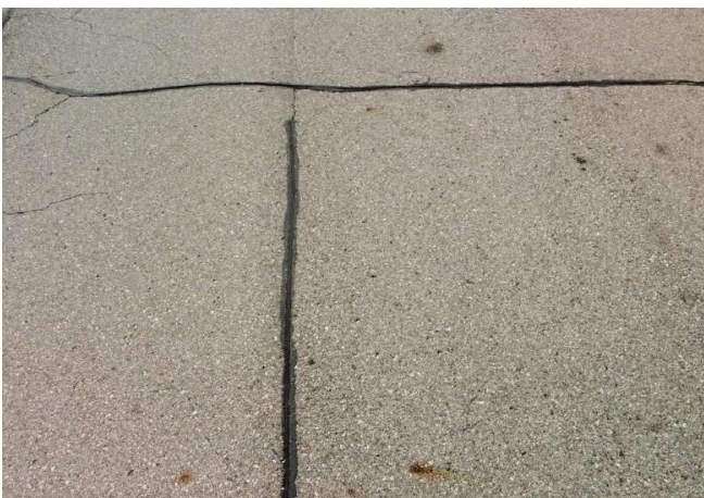
Crack repairs
