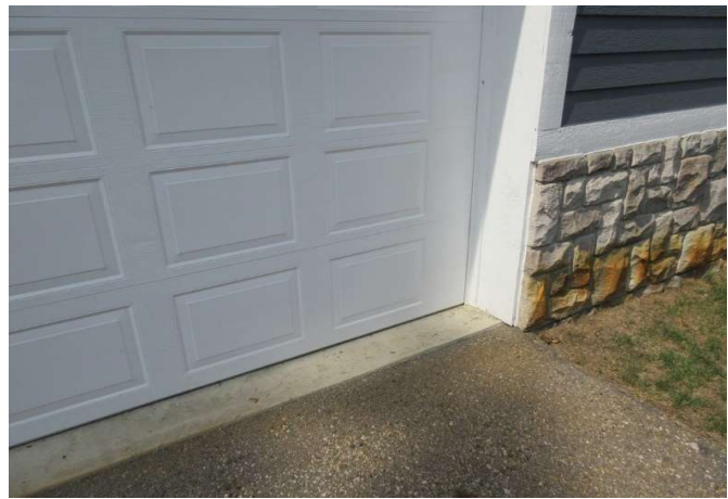
Typical exterior condition
