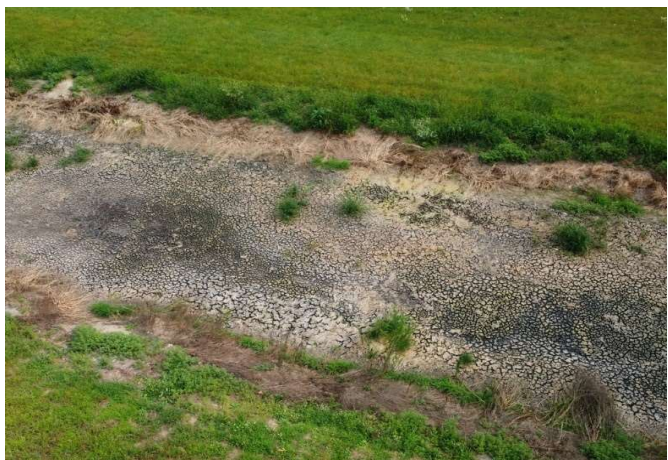
View of leach field
