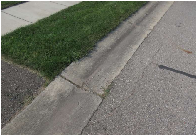
Curb along road
