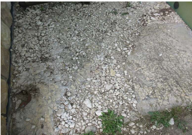
Deteriorated concrete
