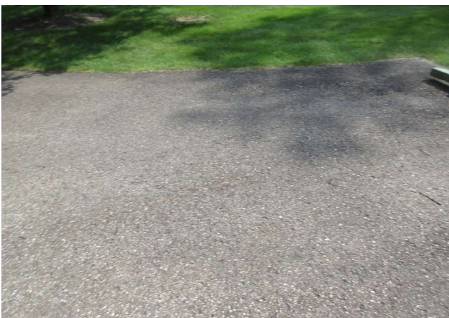
Pavement at wellhouse
