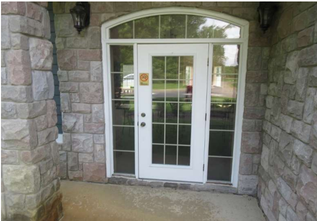
Typical clubhouse entry door
