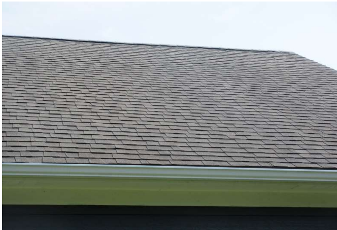
Roof at clubhouse
