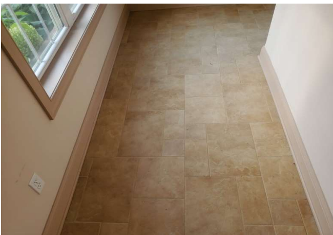
Floor in clubhouse hallway
