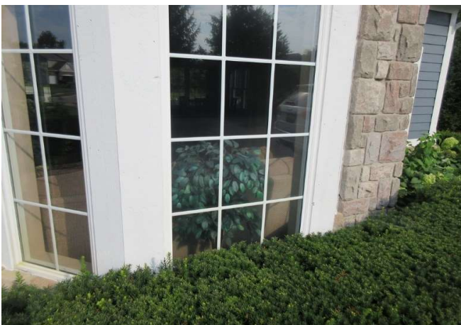
View of bay window
