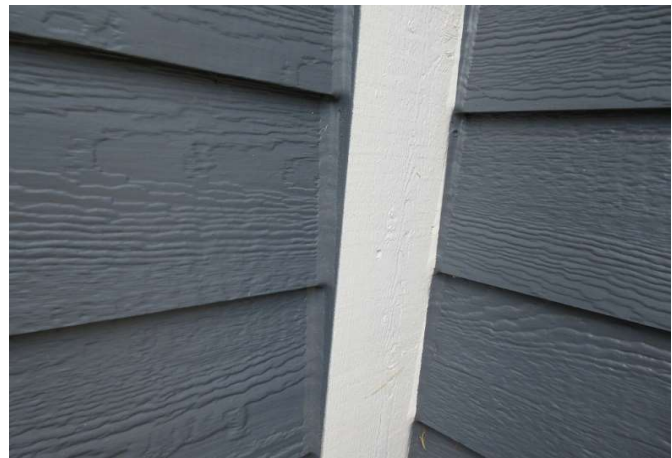
Detail of siding
