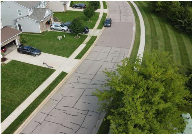
View of road
