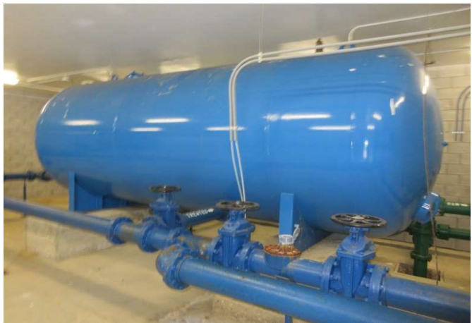
View of water storage tank
