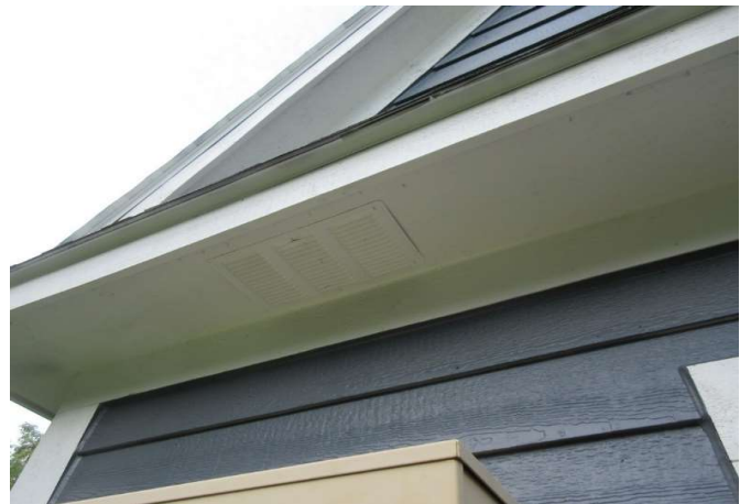
Vented soffit panel and painted surfaces
