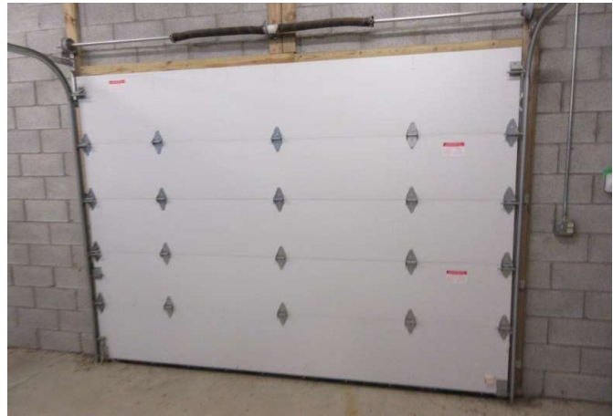
Interior of garage door
