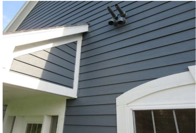
Siding at clubhouse
