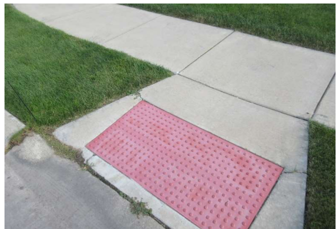
ADA ramp at road
