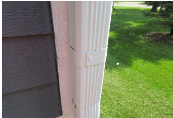
Downspout connection
