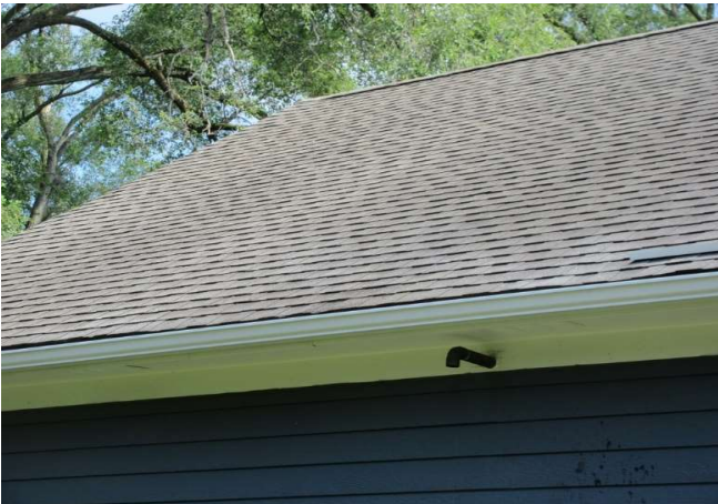
View of shingles
