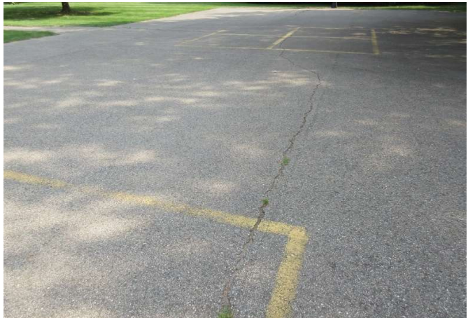
View of asphalt court
