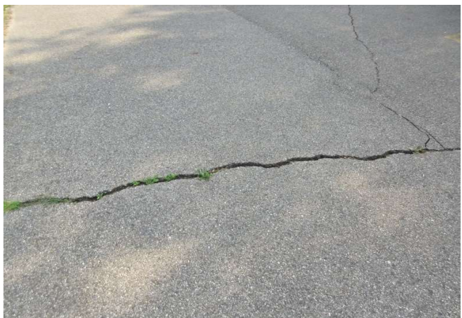
Large crack in play surface
