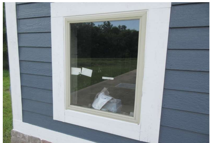
Window at pumphouse
