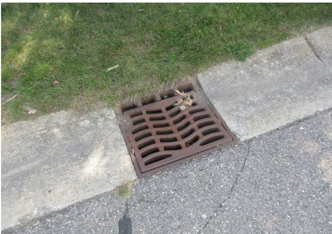
View of inlet grate
