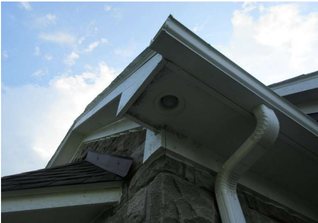
Gutter at soffit
