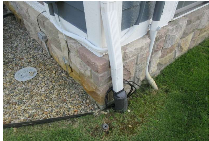
Downspout at grade
