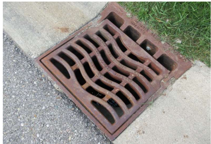
Inlet in curb
