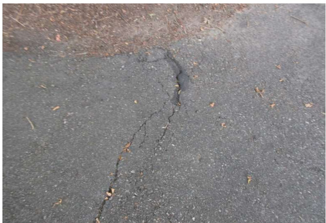
Surface crack
